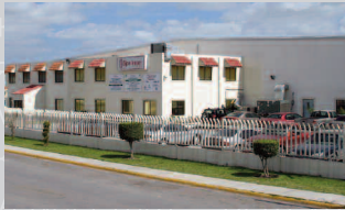
Matamoros, Mexico 88,000-square-foot manufacturing center, mirroring our New York headquarters in capital equipment and production process technologies.
